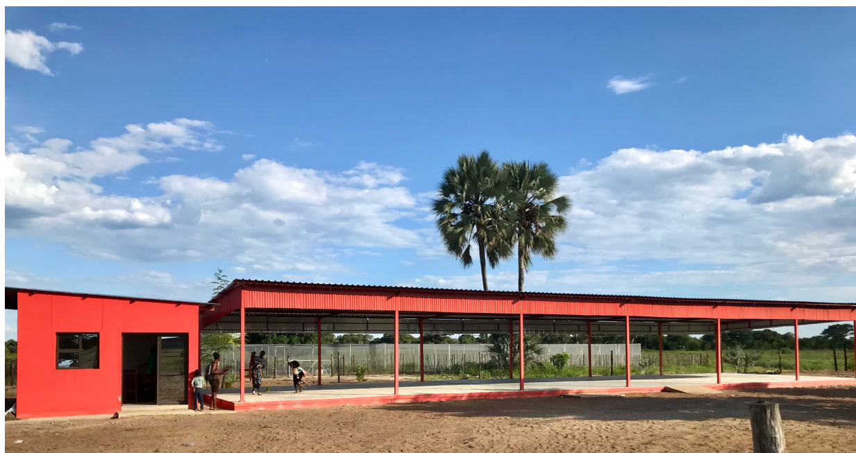
Market place constructed at Ncamagoro Community Forest, Kavango West Region, under the Empower to Adapt project
