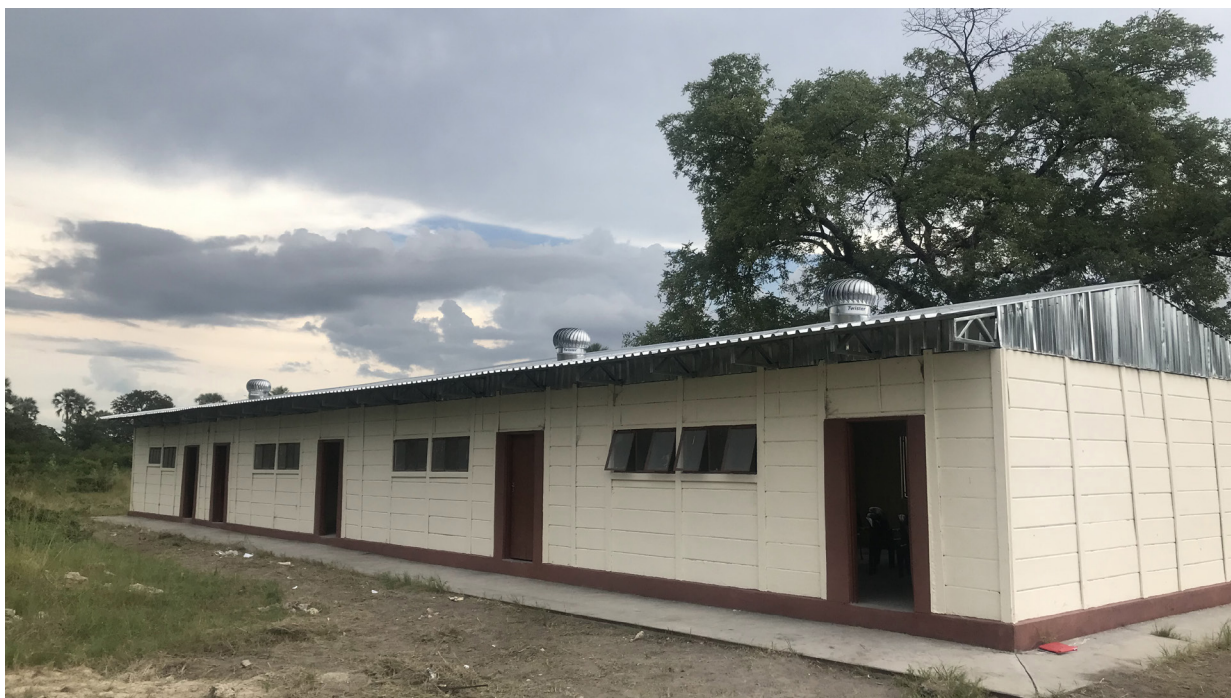
Flood relief centre built at Lusese Conservancy, Zambezi region.
