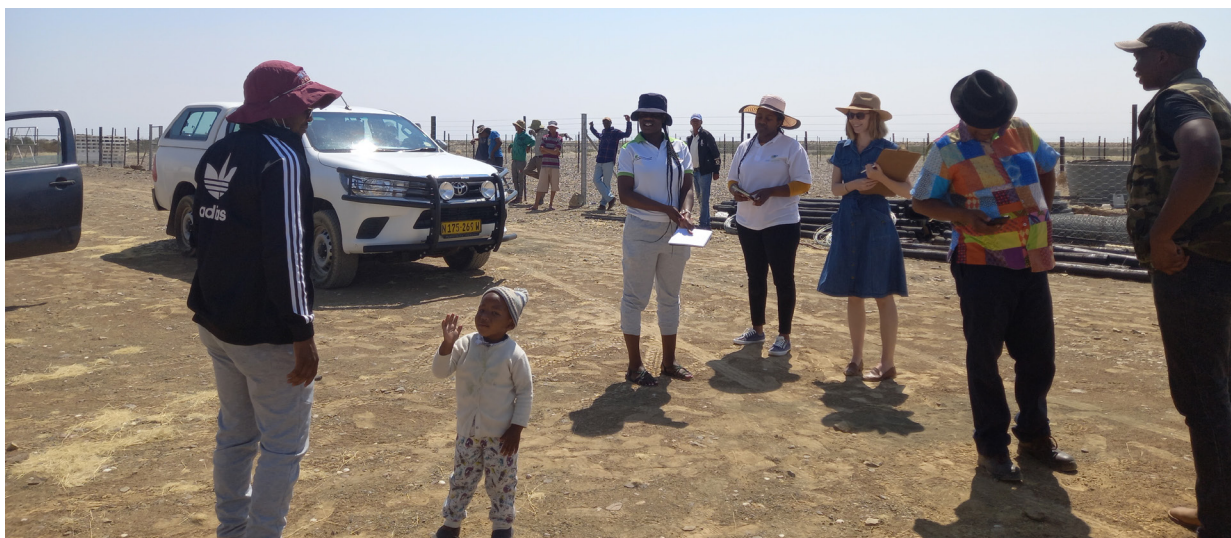
Visiting the site of the feedlot under construction in !Khob !Naub Conservancy, /Karas Region, October 2022
